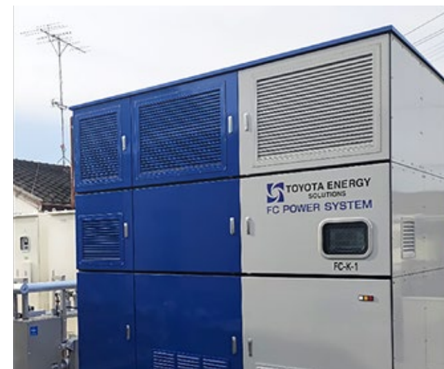
Toyota Energy Solutions' fuel cell generator
