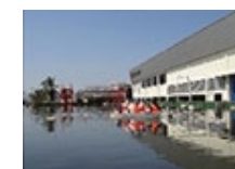
Flooding in Thailand
