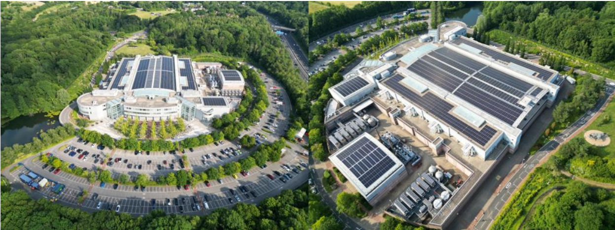
Image 1 – New solar scheme implemented at Swanwick Air Traffic Centre
