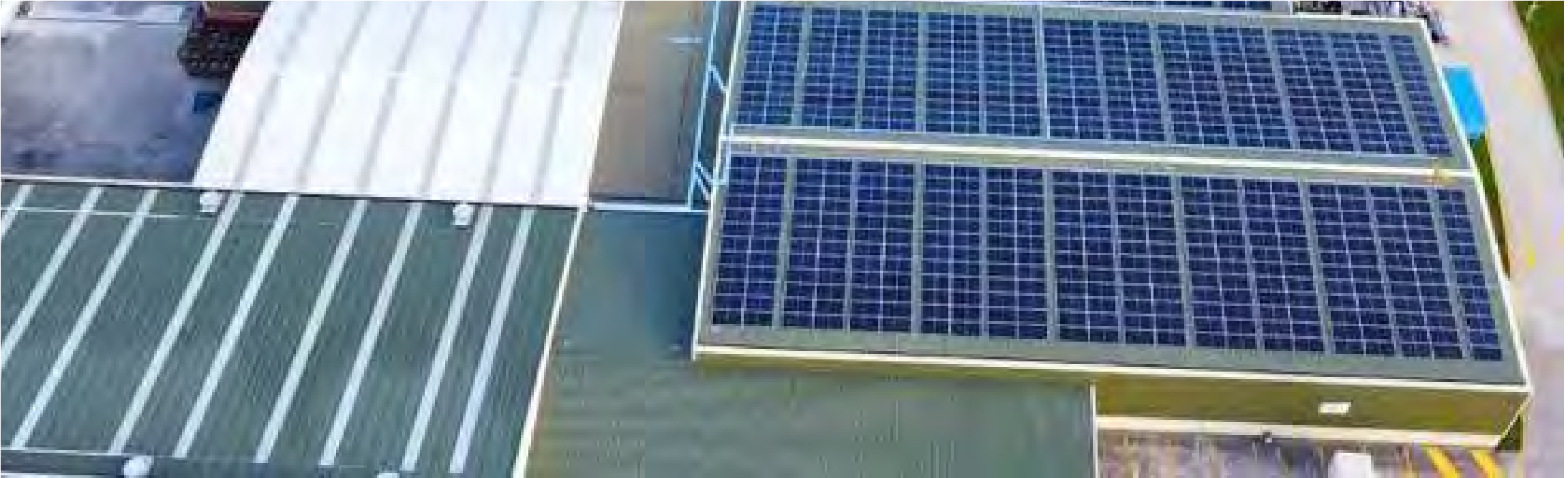
Aerial view of the Carballo self-consumption plant (Spain)
