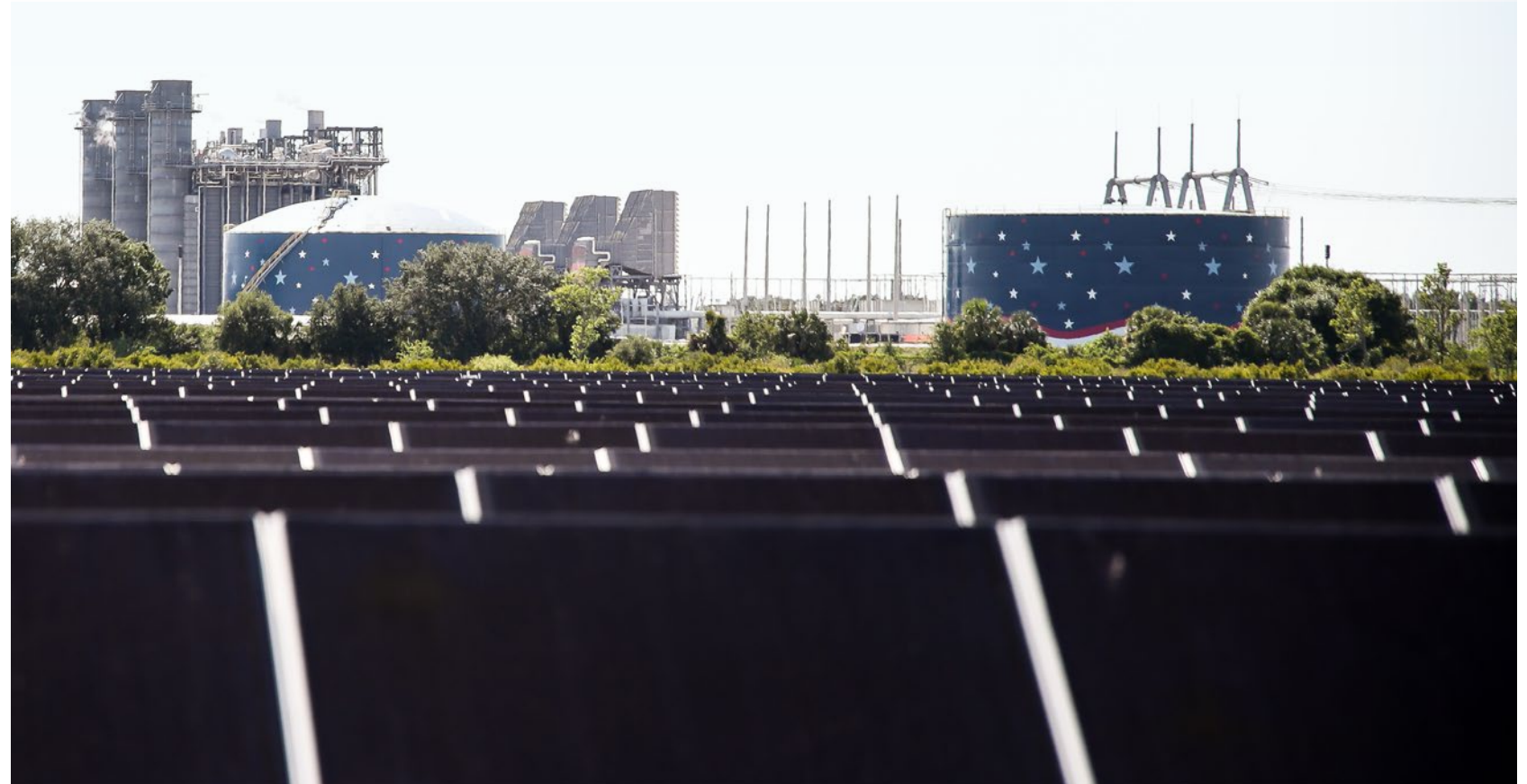
Cavendish Solar Energy Center in Okeechobee, Fla.
