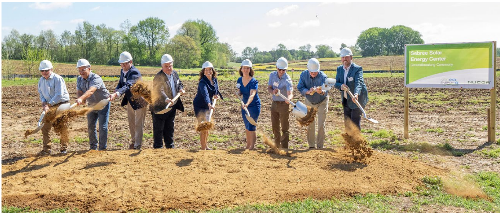
Nucor Corp. representatives and other stakeholders participate in NextEra Energy Resources' groundbreaking for the Sebree Solar Energy Center in Robards, Ky.
