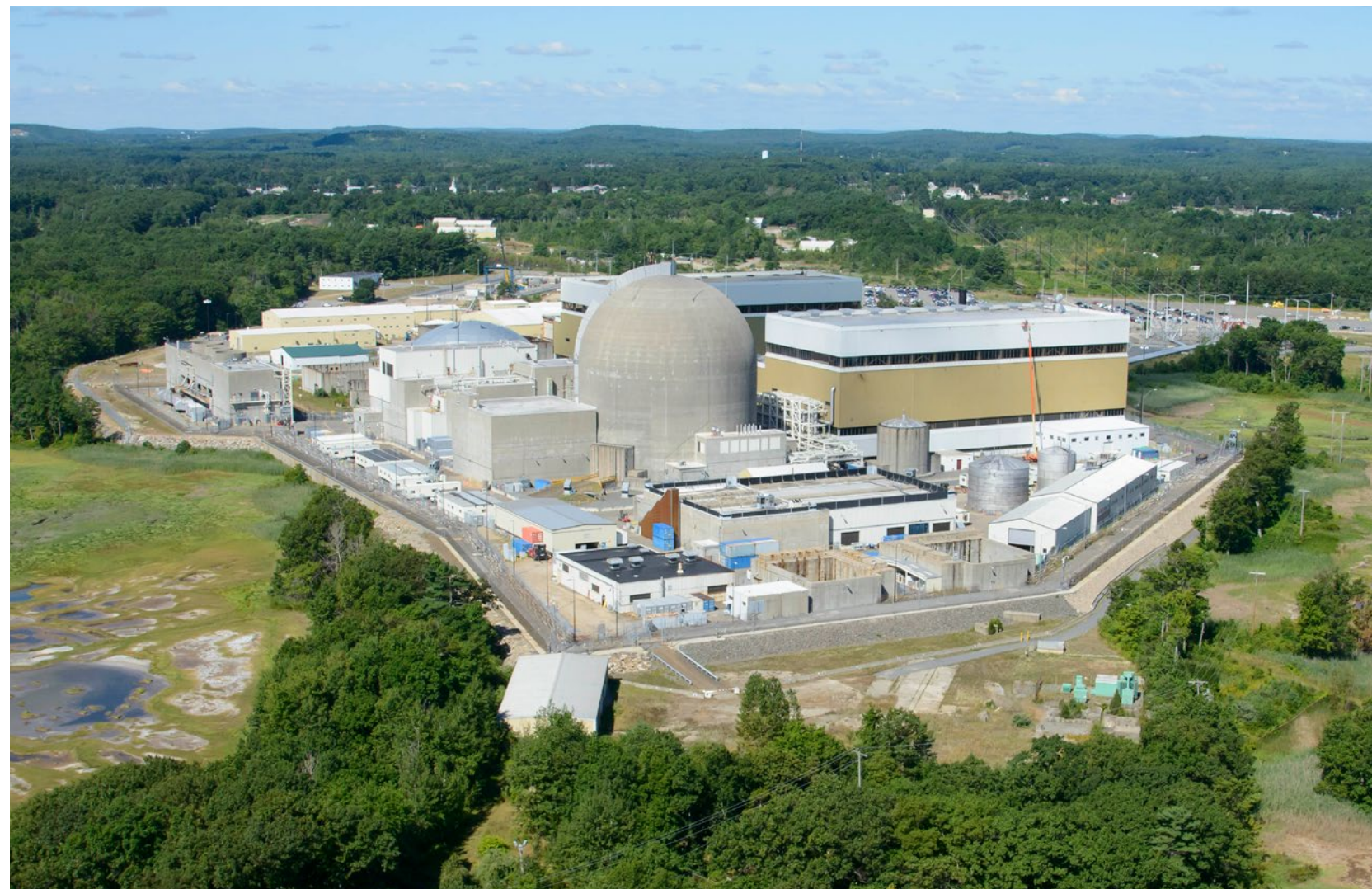
Seabrook Nuclear Power Plant in Seabrook, N.H.
