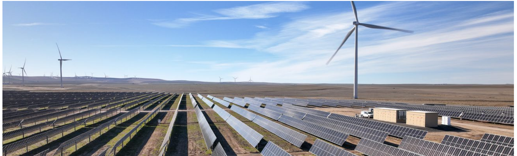
Wheatridge Renewable Energy Facility in Heppner, Ore.
