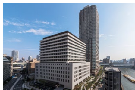
Exterior view of the new hospital
