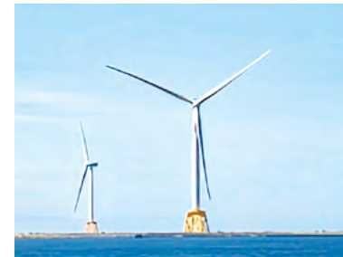
Wind power generation (at bottom is the jacket foundation), source: Ishikari City HP
