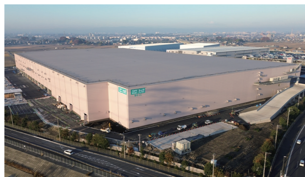
Exterior of Satte DC
