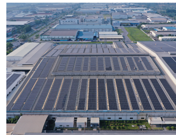
Solar power generation at Hanoi Factory
