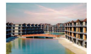
1st district exterior photo
