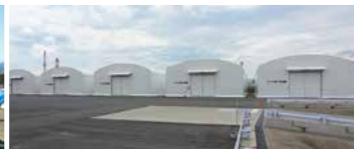
2023 Land leveling work is completed
