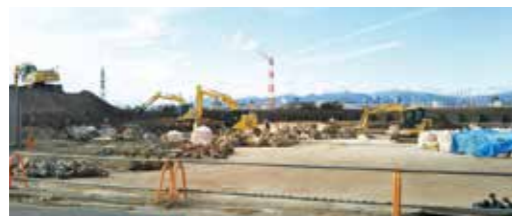
2018 Removal work is underway
