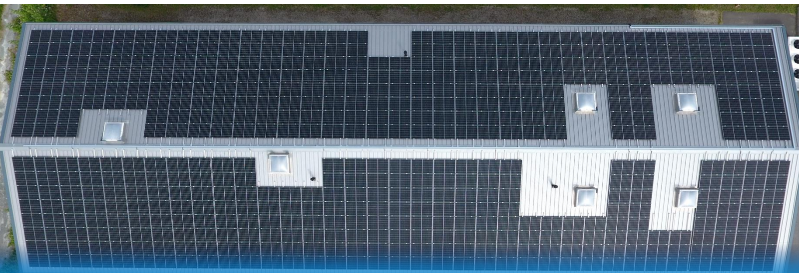
Solar panel installation at Neo's facility in Sagard, Germany.
