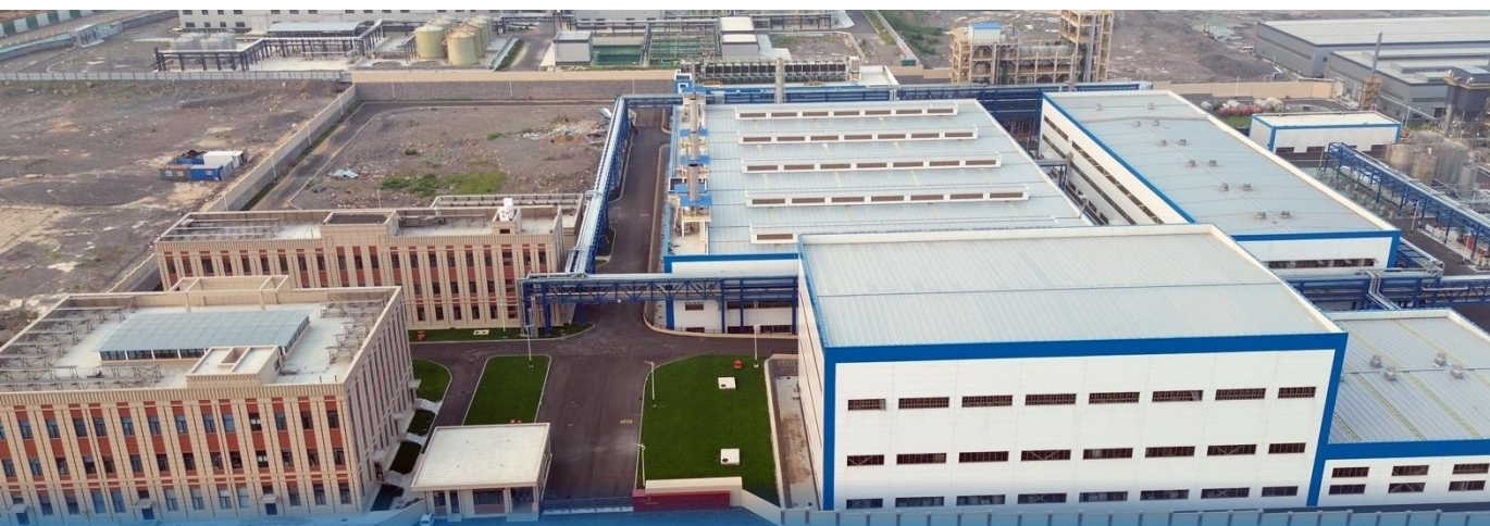
Solar panels are installed at Neo's emission control catalyst facility in Zibo, China.
