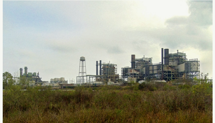
689 MW natural gas combined cycle unit at NRG's Cedar Bayou plant
