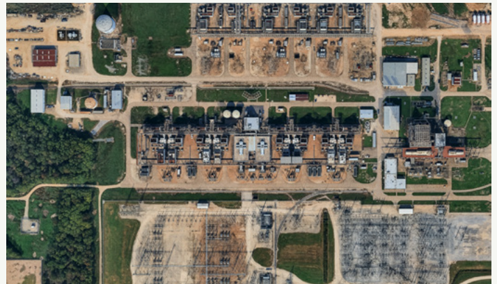
415 MW quick-start natural gas peaking project at NRG's TH Wharton plant
