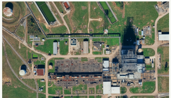
443 MW quick-start natural gas peaking project at NRG's Greens Bayou plant
