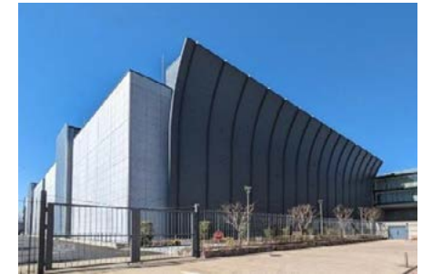
Mitaka Data Center EAST
