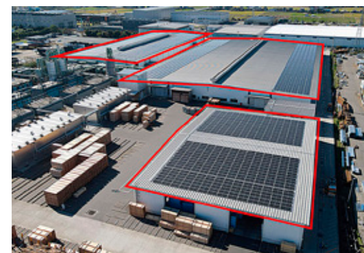
Cypress Sunadaya Toyo Industrial Park factory. Red marks show the solar power-generating equipment
