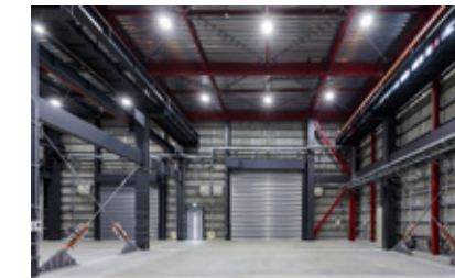
Inside of the Open Lab 3 (red steel frames are used materials and black steel frames are new)
