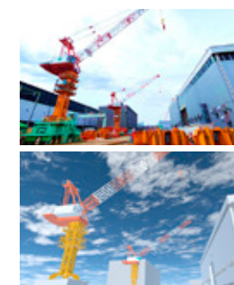
A digital twin: (above) Real construction site, (below) digital twin cyberspace
