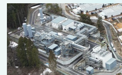
Sabatier methanation demonstration facility (under construction)
