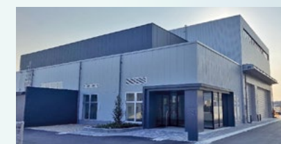
SOEC methanation bench-scale test facility (Completion in June 2025)
