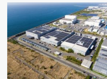
Photovoltaic power generation systems at Nishikinohama Factory, Panasonic Energy
