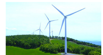
An onshore wind power generation plant for the Panasonic Group.
