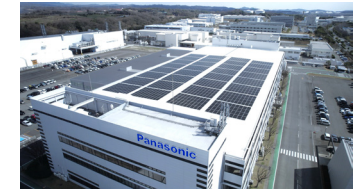
Photovoltaic power generation systems at Kobe Factory, Panasonic Connect Co., Ltd.
