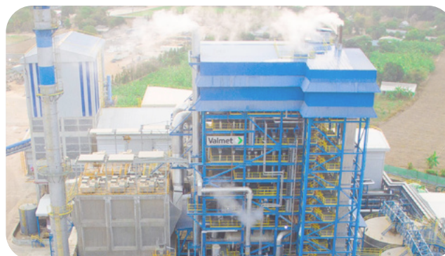
Recovery boiler Thai Paper Co., Ltd. (Pulp Production-Wangsala).
