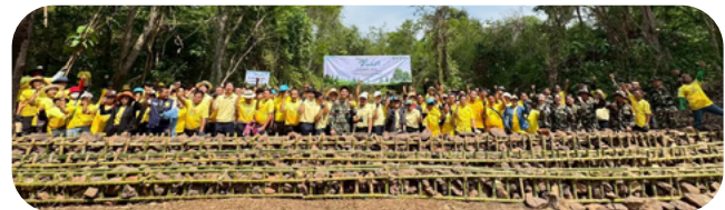
Check dam construction projects - Khon Kean.
