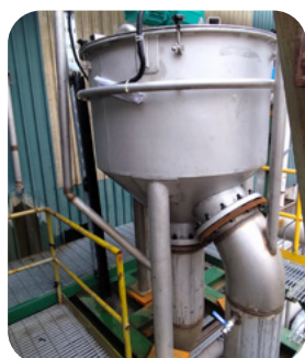
Reused water - Fine filtration, PT Fajar Surya Wisesa Tbk.
