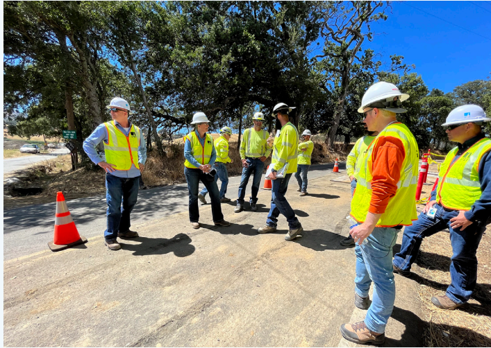
Patti Poppe (second from left) visits crews at an undergrounding project site in Fairfield, Calif., aimed at protecting customers from wildfire and other climate-driven events.
