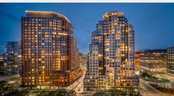
The Grace and Reva, a residential and mixed-use complex in the National Landing submarket of Arlington, Virginia
