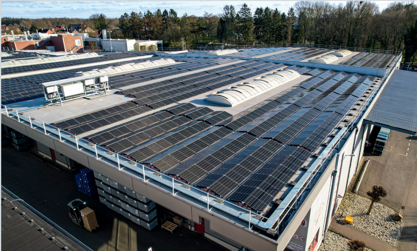
The 2,500 solar modules on the rooftops of the POLYTEC plant in Lohne could supply roughly 250 households with electricity.
