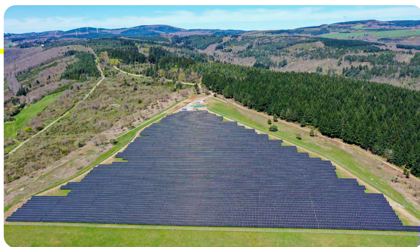
Aerial View of La Gineste, France (Copyright: AbsoluDrones)
