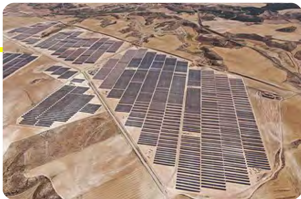
Example solar park by QENERGY in Spain (Copyright: QENERGY)
