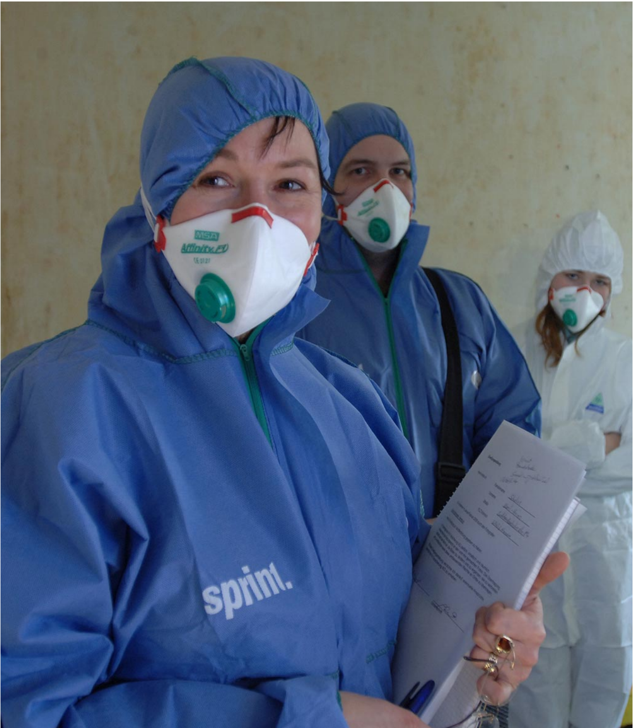
Employees of the R+V restoration specialist Sprint at work in a damaged building.
