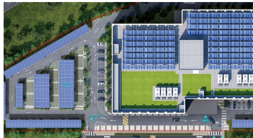
Solar Power Installations at Dongtan Data Center
