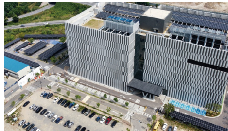
Panoramic View of Dongtan Data Center
