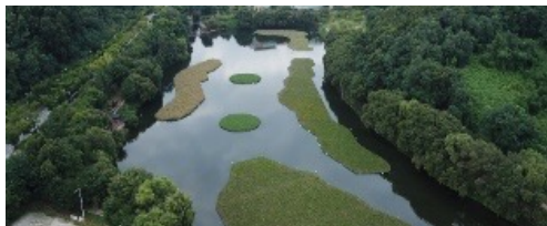
Installing ecological plant islands for reservoir management
