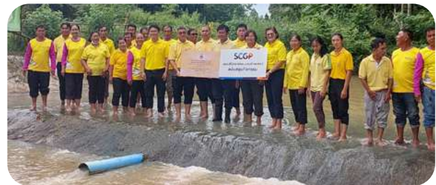
SCGP supports the construction of a cement check-dam in Khon Kaen Province, 2024.
