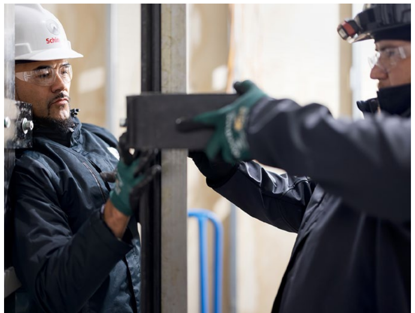
Ikaika Thomas and Alan Espinoza installing crossbeams.
