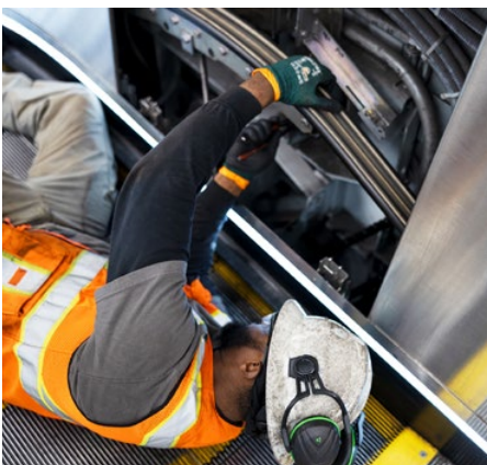
Robert Johnson (above) and Chandler Rosselle (right) working in confined spaces.
