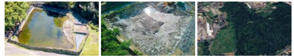
H:H Dam before rehabilitation
