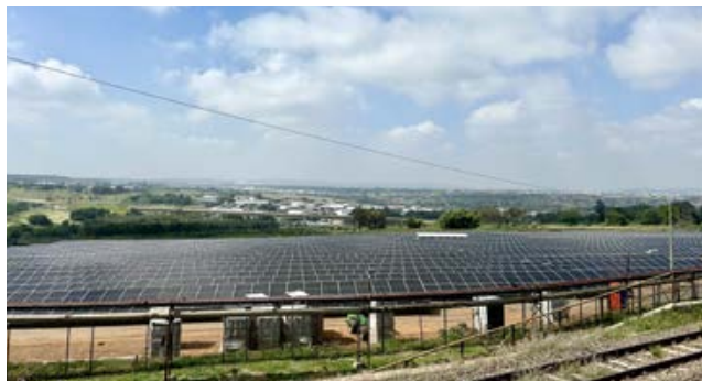
Modderfontein solar park installation, Johannesburg, South Africa
