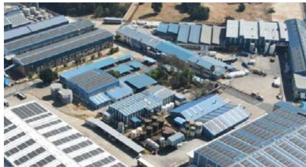
Chempark rooftop solar project, Johannesburg, South Africa
