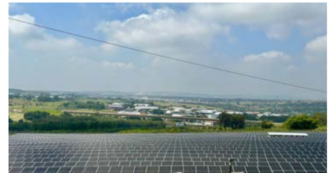
Modderfontein solar park installation, Johannesburg, South Africa
