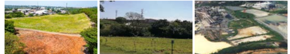
H:H Dam after rehabilitation
