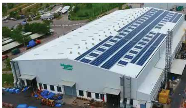
Schneider Electric's factory for transformers and medium and low voltage switch gear in Vadodara India generates approximately 1 GWH per year of onsite solar electricity
