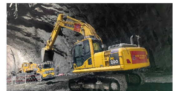
Application of a remote control intelligent excavator
