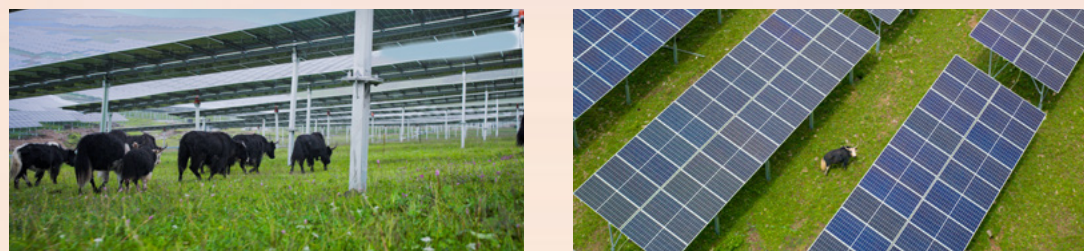
Yaks Pass under the Solar Power Panels of Kela Solar Power Station Phase I
