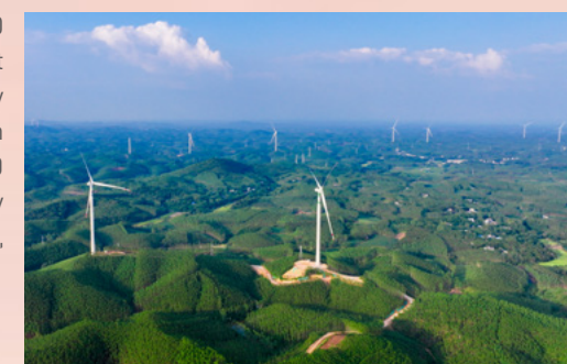
Nasi Wind Farm of SDIC Guangxi New Energy in Qinnan District
