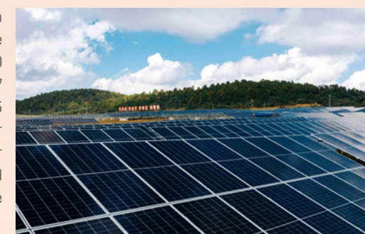
Zhalashan Solar Power Project on the Yalong River under construction
