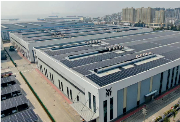
Solar panels in Yuhan, China
