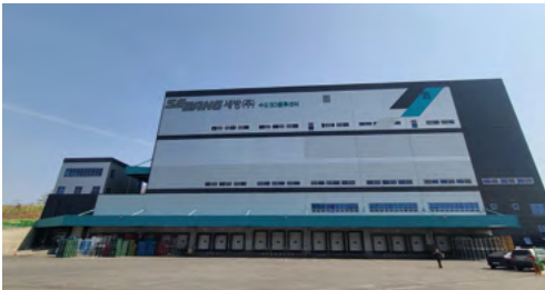
Metropolitan 3rd Logistics Center
