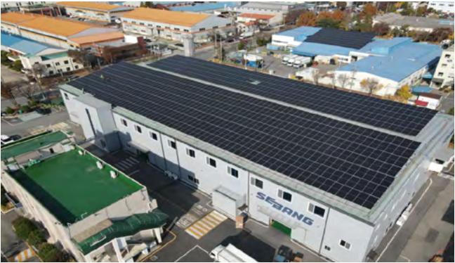
SOLVIC Unit 10 Solar Power Plant (PV: 499.59kW) Installation location: 236 Sonjae-ro, Gwangsan-gu, Gwangju Commercial operation date: 2025.01.21
