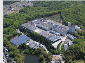
Hyogo Factory mega solar
