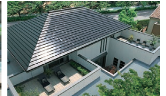
Sekisui House proprietary tile-shaped photovoltaic panels
