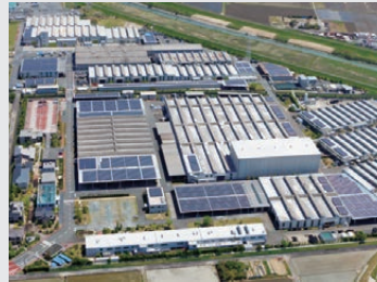
Shizuoka Factory mega solar
