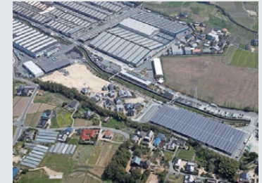
Yamaguchi Factory mega solar
