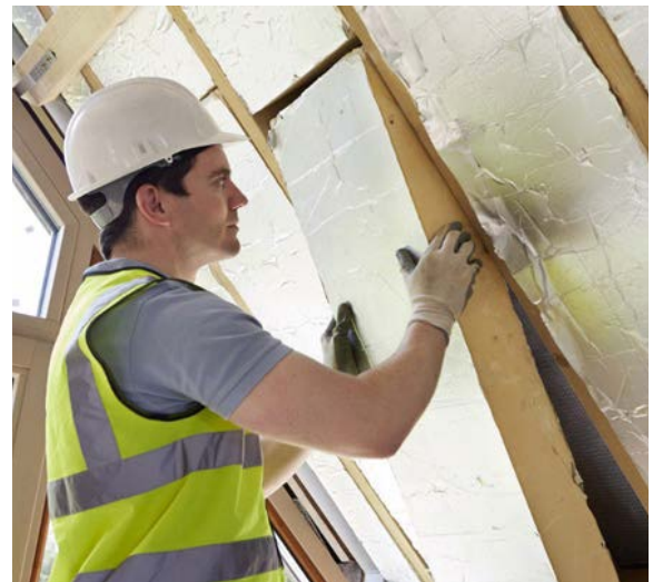
Installing insulation boards. Photo credit: edie newsroom
