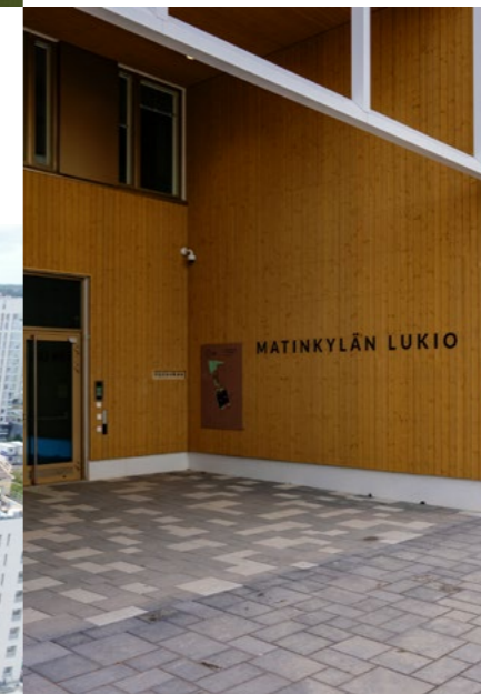
Matinkylä upper secondary school and swimming pool NPS 100 (handover phase)
