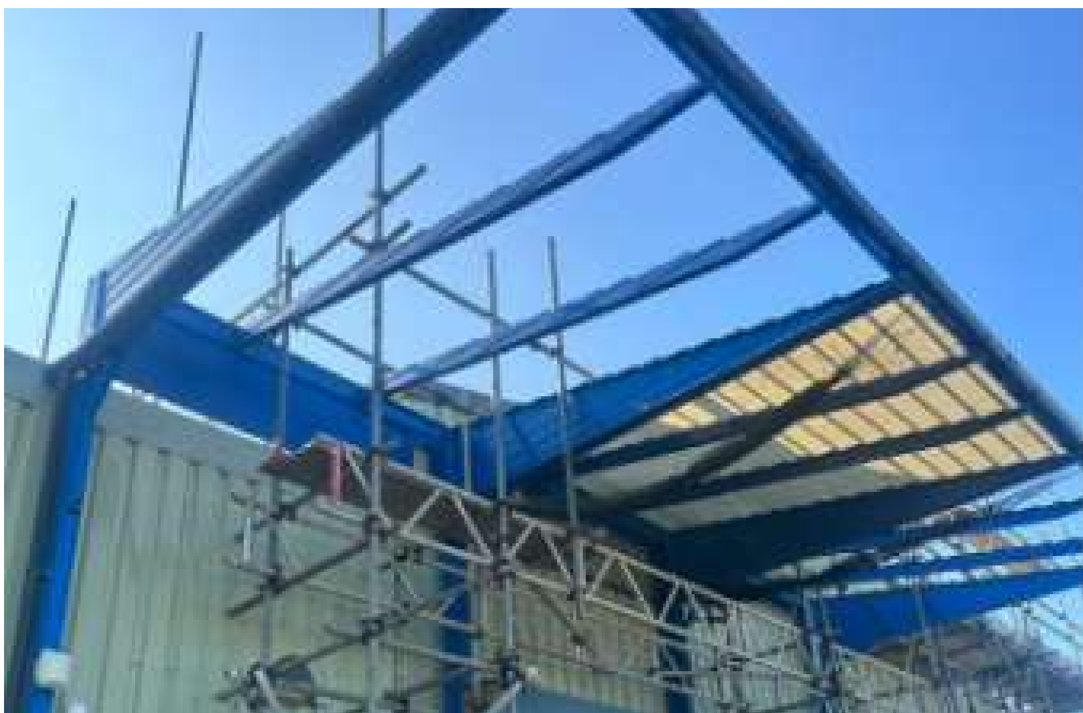
Bottom Left: Replacing an asbestos roof
