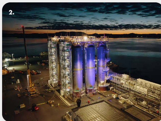
1, 2. The Northern Lights receiving terminal in Norway. CO 2 is transported by ship, then piped 100 km offshore and stored 2,600 metres under the North Sea.
