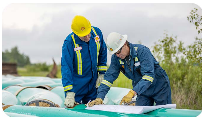
Photo: Shell Canada Integrated Gas employees at work on a pipeline project, Fort St. John, British Columbia.
