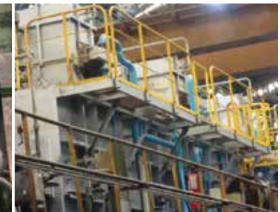
CG1 1JC cooling fan improvement
