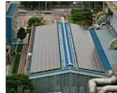
Rooftop solar power system installation project
