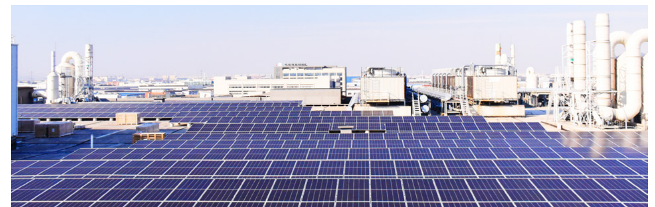
▲ Wuxi SCC and Nantong SCC's photovoltaic panel installation capacities each reach 4 megawatts
