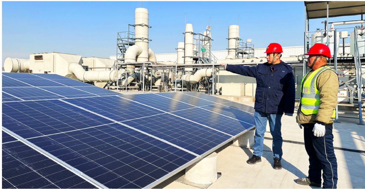
▲ Li Tiejun is conducting an inspection with suppliers on the newly installed photovoltaic panels
