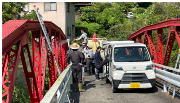
Bridge maintenance activities
