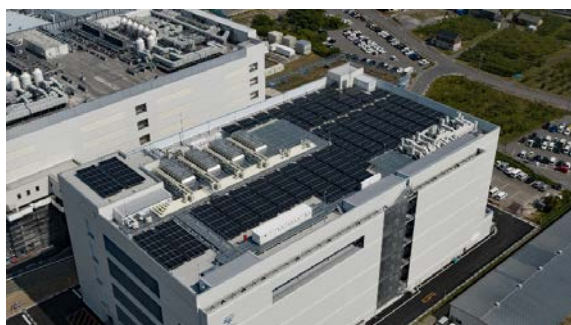
(Takaoka Plant (Nakano City, Nagano Prefecture) Building E)
