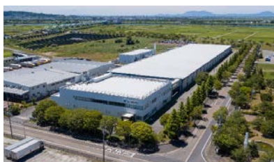
Kyogase Plant (Agano City, Niigata Pref.)
