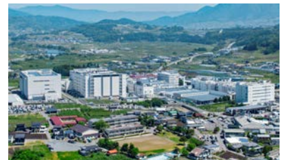
Takaoka Plant (Nakano City, Nagano Pref.)
