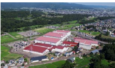
Arai Plant (Myoko City, Niigata Pref.)
