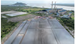
Facilities of Chitose Laboratory Corp./NEDO (New Energy and Industrial Technology Development Organization)
