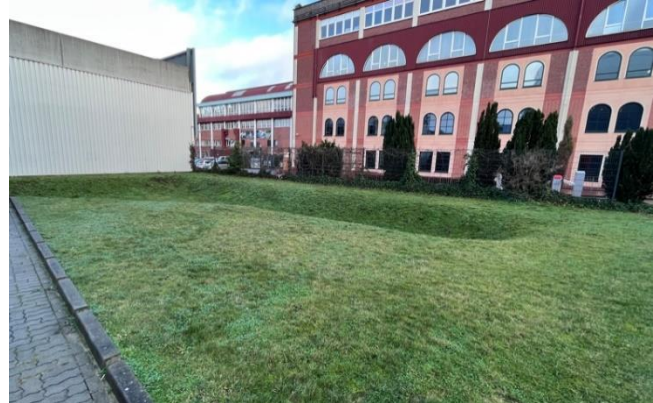
Water retention area created on our plot of land in Wandsbek.
