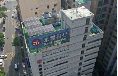
The rooftop solar PV system at Bank SinoPac Beigao building.
