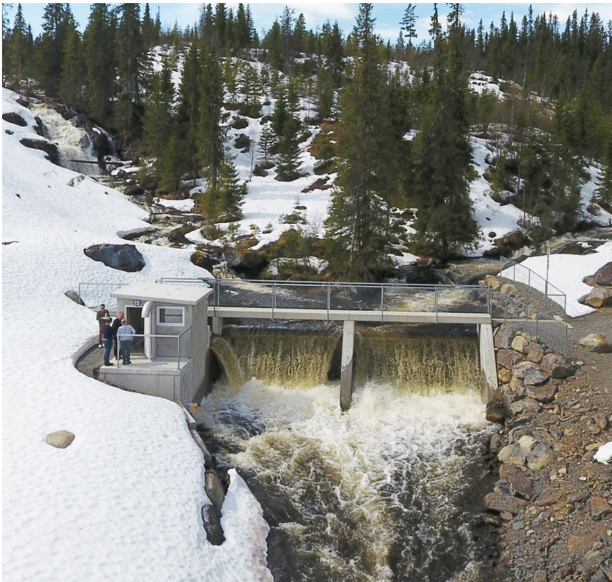
The intake for the Liaelva power plant in Sør-Aurdal municipality, Innlandet county.
