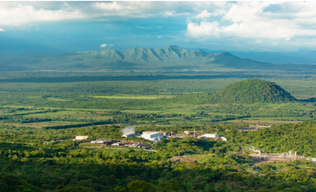
Geothermal project in Nicaragua
