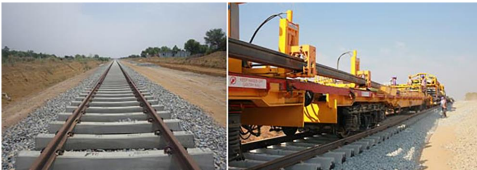
At the track laying site
