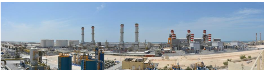
[Mirfa power and desalination plant]
