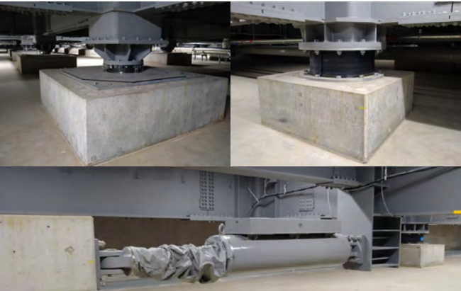
Hybrid seismic isolation structure
