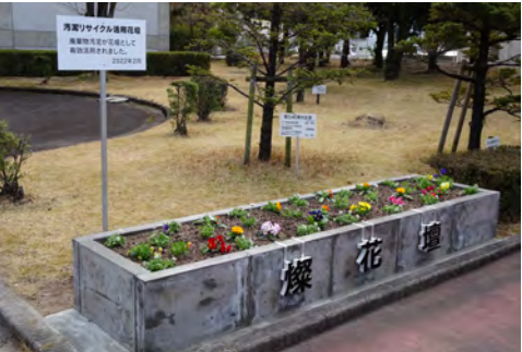
Flowerbed made from blocks of recycled sludge
