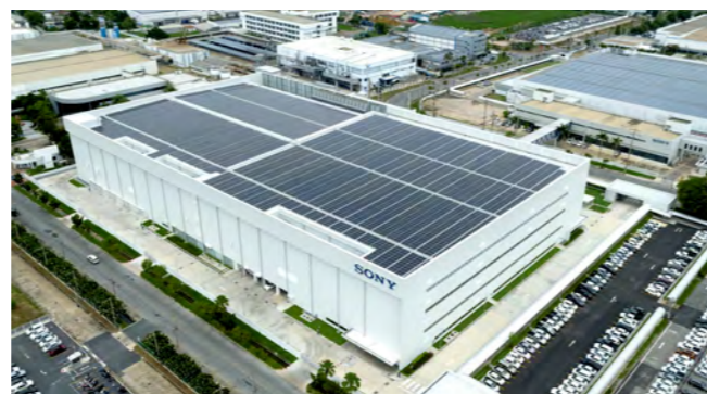
Solar panels at the SDT's new building
