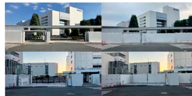
Waterproof walls of the main gates and south gates
