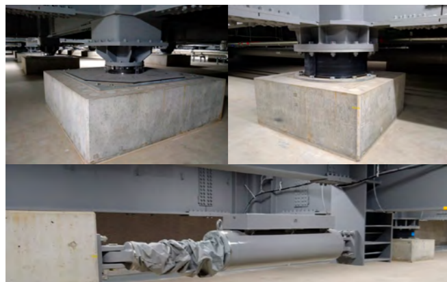
Hybrid seismic isolation structure
