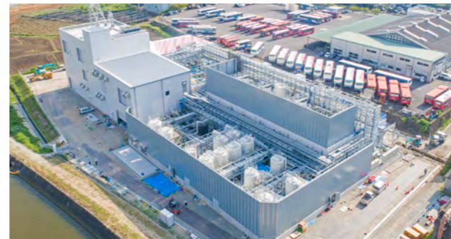
The sewage treatment facility of Nagasaki TEC
