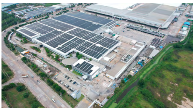
Solar panels at STT
