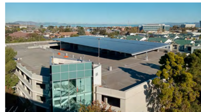
Solar panels at Sony Interactive Entertainment San Mateo
