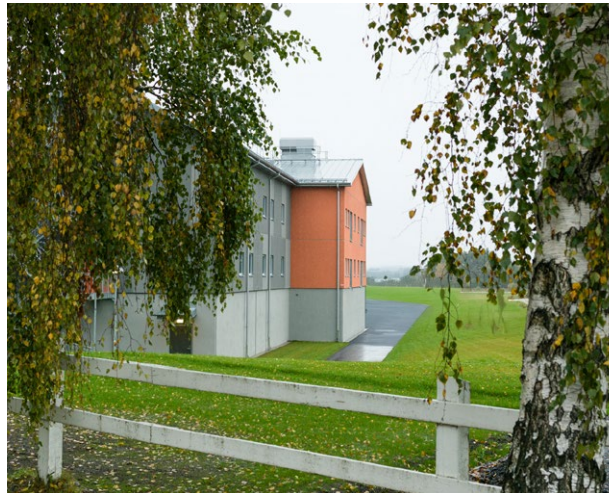
One of the many construction projects completed during the year was the new accommodation block at Rödjan correctional facility; read more on page 24.
