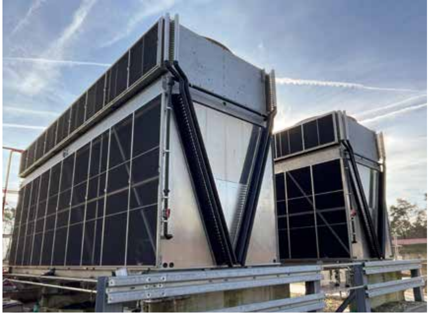
Since as early as 2011, Storck has been using hybrid recoolers, which require about 35% less energy than alternative systems.
